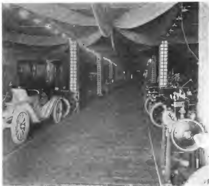
Looking North on an Aisle on the Second Floor
